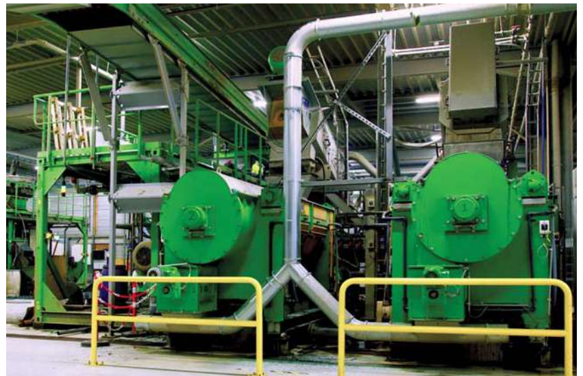
Figure 3 – Washing facility for shredded geotextile material to remove embedded soil (Groen & Gruber, 2025).
