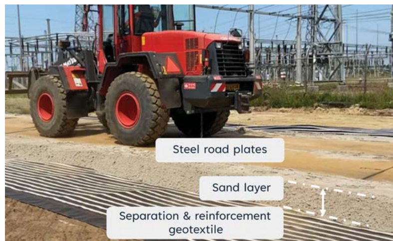
Figure 1 – Example structure of a temporary construction road using a geotextile.
