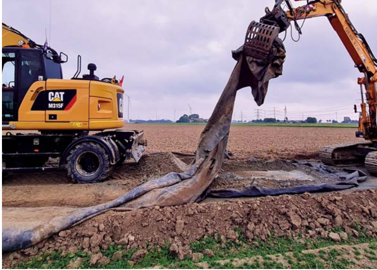
Figure 3 – Removal of a temporary construction road.
