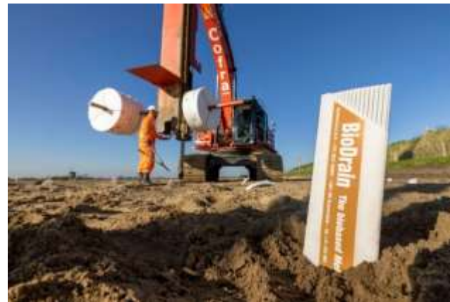
Verticale drainage biobased polymeer
