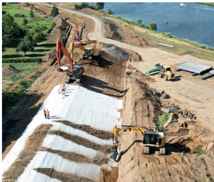
Figure 6 – Cross-section of a levee for flood protection with geosynthetics.
