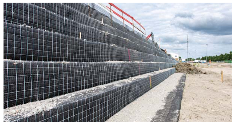
Figure 1 & 2 – Reinforced slope A24, Blankenburg connection, Rotterdam. Steep slopes, longer embankment resulting in considerable saving in concrete.
