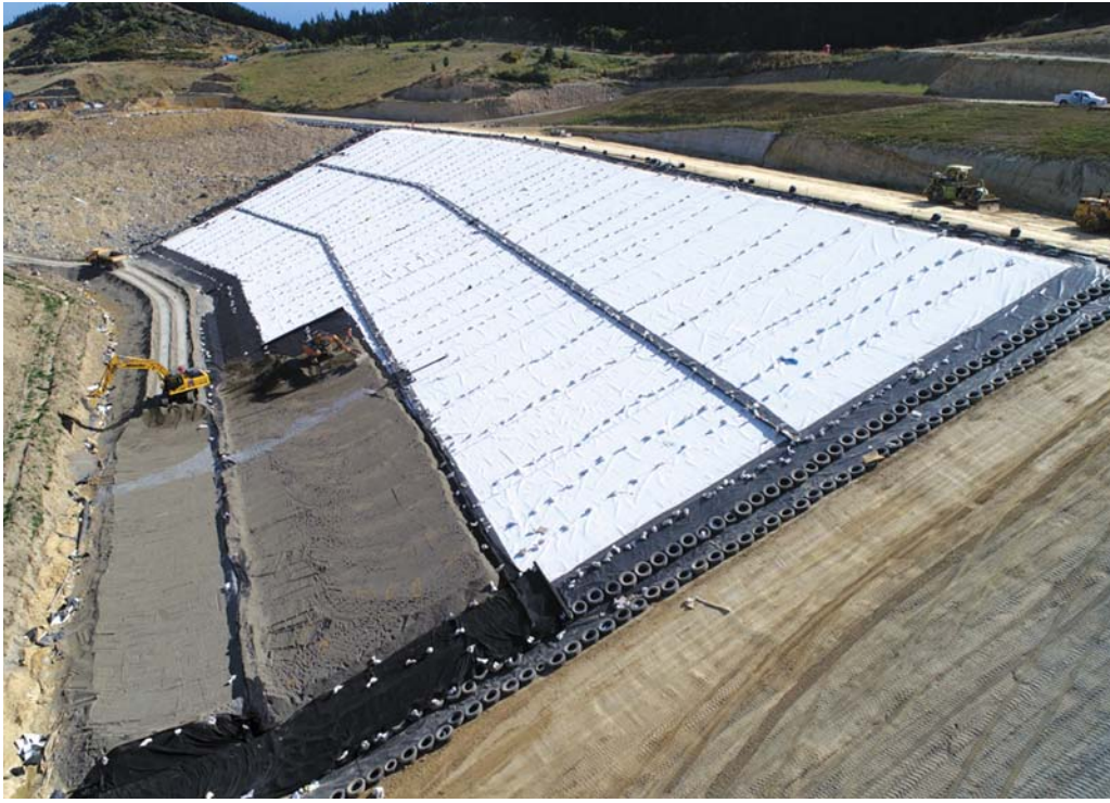
Figure 4 – Example using geosynthetics in landfills with geomembranes and drainage mats by Boyd Ramsey.
