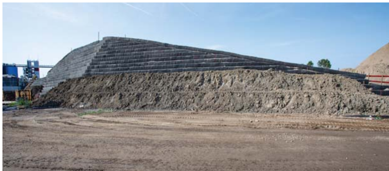
Figure 1 & 2 – Reinforced slope A24, Blankenburg connection, Rotterdam. Steep slopes, longer embankment resulting in considerable saving in concrete.
