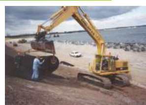
Reinforced grass in higher part of the slope of a dike, Zeeland
