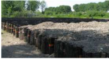
Platform under construction site of wind turbine, Vlaardingen
