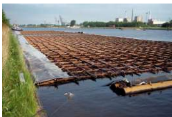
Fascine mattress with filterlayer in bottom protection, Rotterdam
