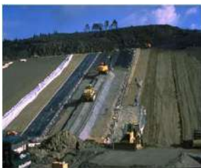
Anchorage of veneer-layer on landfill cover
