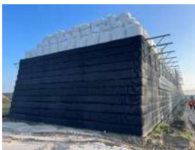
Reinforced slope, Moerdijk
