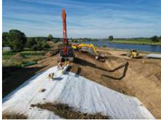
Bentonite mat instead of clay on top and outside slope , Beesel
