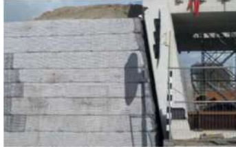
Earth pressure relief structure behind concrete wall, without connection
