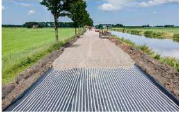
Reinforcement of roadfoundation
