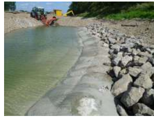
Geosynthetic tube as artificial island
