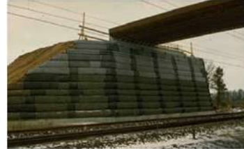
Earth pressure relief structure behind concrete wall, without connection
