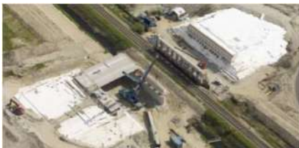
Light weight ramp of viaduct over railway line Alphen a/d Rijn - Gouda
