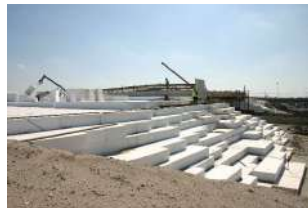
Light weight ramp of viaduct over railway line Alphen a/d Rijn - Gouda
