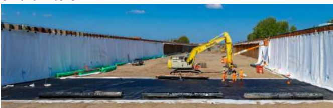
Open tunnel with geomembrane and nonwoven protection layer, N 206, Katwijk
