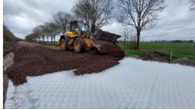
Geocells as base reinforcement
