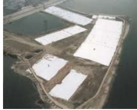
Reclamation IJburg, Amsterdam
