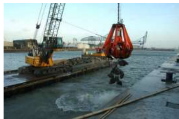
Fascine mattress with filterlayer in bottom protection, Rotterdam
