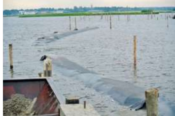
Geosynthetic tube as artificial island
