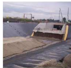
Access road to tunnel
