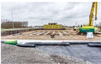
Pile-supported geosynthetic mattress, A4 Hofvliet, Leiden
