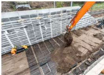
Anchored reinforced wall, Steenwijkerland
