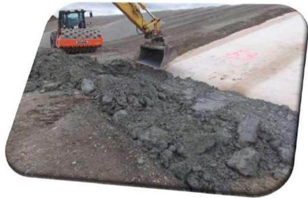
GCL anchoring in the clay core
