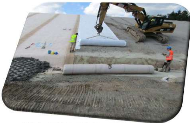
GCL installation wit 0.5m overlaps Placement of geosynthetic drainage mat
