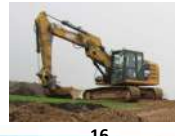
16 Cover soil placement
