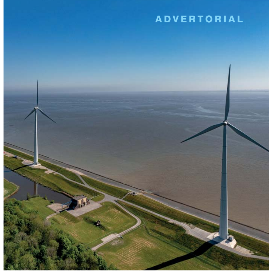
Windfarm Oosterpolderdijk (Credits: RWE)
