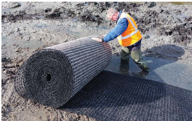
Figure 7 – Installation of a reinforced High Performance Turf Reinforcement Mat (HPTRM) for slope protection.
