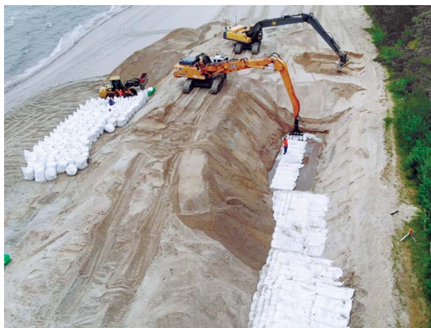
Figure 6 – Installation of Geotextile Sand Containers (GSCs) as a coastal protection measure in the dune core of the sandy beach, Ludmin, Germany.
