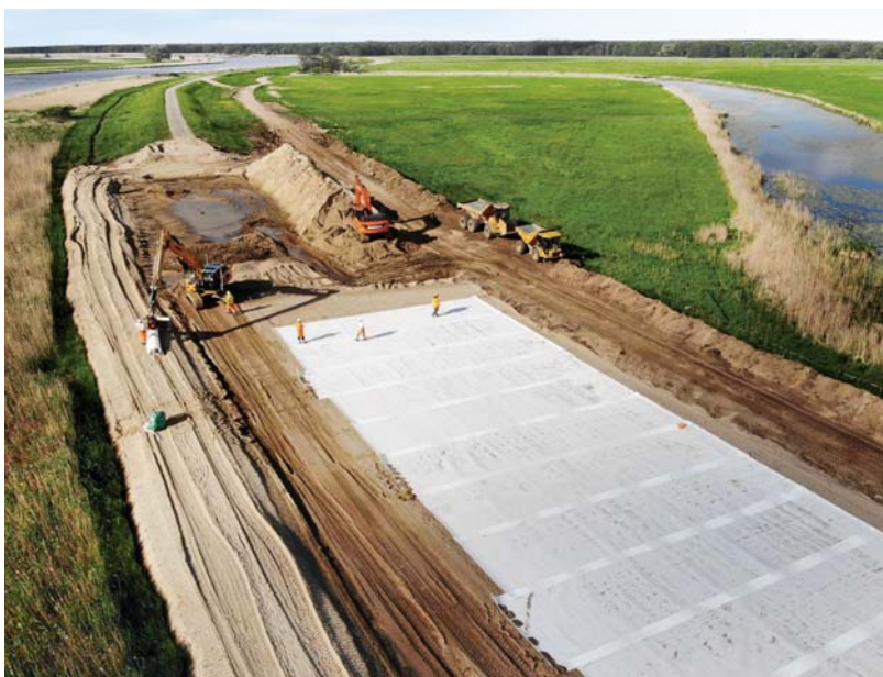
Figure 8 – Installation of high strength geogrids as basal reinforcement below the flood defence at the Oder, Germany.
