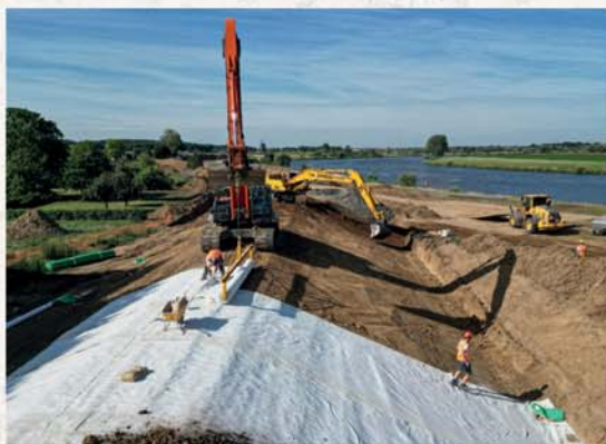
Levee reinforcement Beesel with the installation of geosynthetic clay liner (GCL) on the crest and slopes of the flood defence, replacing a 1 metre thick waterproofing natural clay layer (Waterboard Limburg, contractors Mourik Infra and FL).
