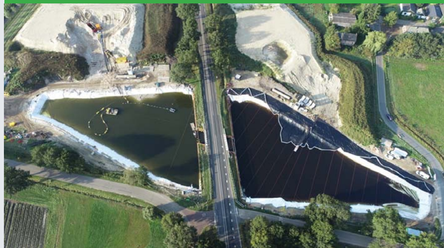
Geomembrane structures for four tunnel ramps "in wet conditions."
