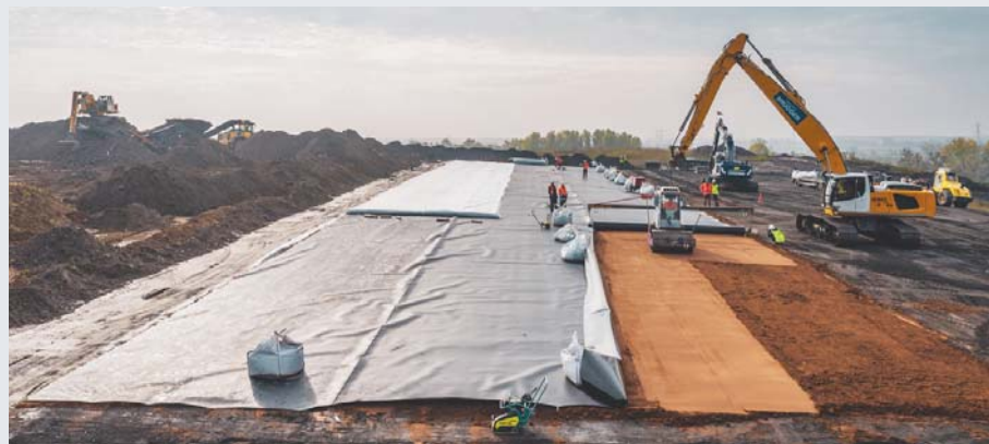
Final closure system of landfill site Derde Merwedehaven Dordrecht
