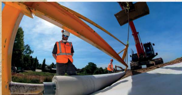
Levee reinforcement Beesel with the installation of geosynthetic clay liner (GCL) on the crest and slopes of the flood defence, replacing a 1 metre thick waterproofing natural clay layer (Waterboard Limburg, contractors Mourik Infra and FL).
