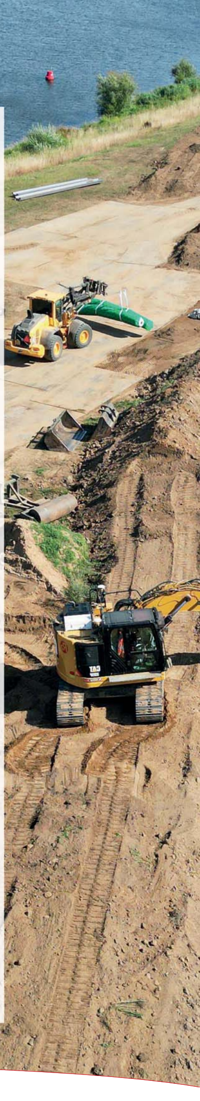
Levee reinforcement Beesel with the installation of geosynthetic clay liner (GCL) on the crest and slopes of the flood defence, replacing a 1 metre thick waterproofing natural clay layer (Waterboard Limburg, contractors Mourik Infra and FL).
