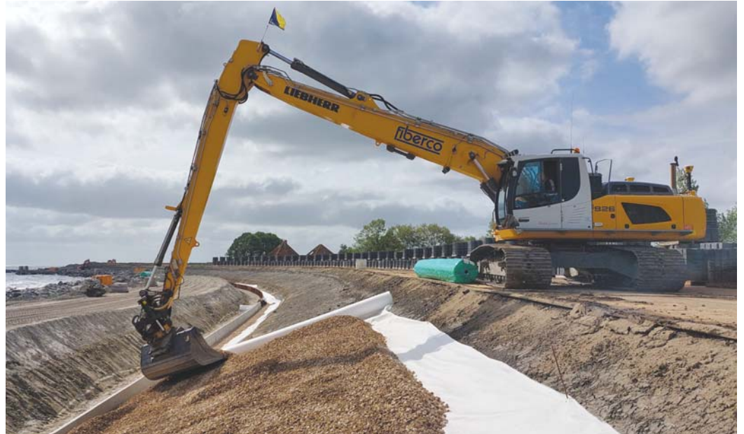
Figure 3 – Filter construction using a non-woven geotextile below a placed block revetment on the slope and rock in the levee toe (Markermeerdijken, The Netherlands).
