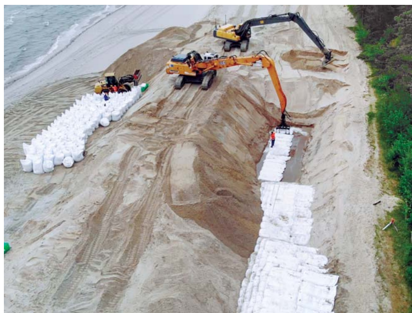
Figure 6 – Installation of Geotextile Sand Containers (GSCs) as a coastal protection measure in the dune core of the sandy beach, Ludmin, Germany.
