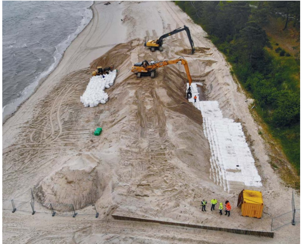
Figure 3 – Construction process of a structure with Geotextile Sand Containers as underground coastal protection measure in the dune core of the sandy beach behind.
