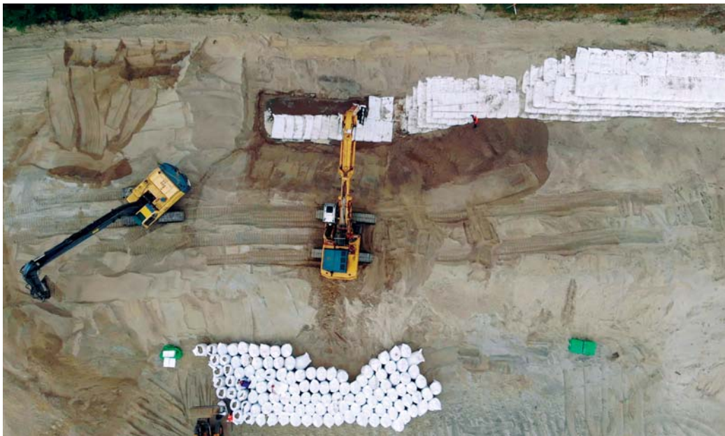
Figure 1 – Construction process of a structure with Geotextile Sand Containers, filled with local beach sand – and installed as an underground coastal protection measure in the dune core of the sandy beach behind.
