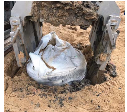
Figure 3 – Installation of Geotextile Encased Sand Columns (GEC) as soil improvement technique for the very soft soil conditions to create bearing capacity.
