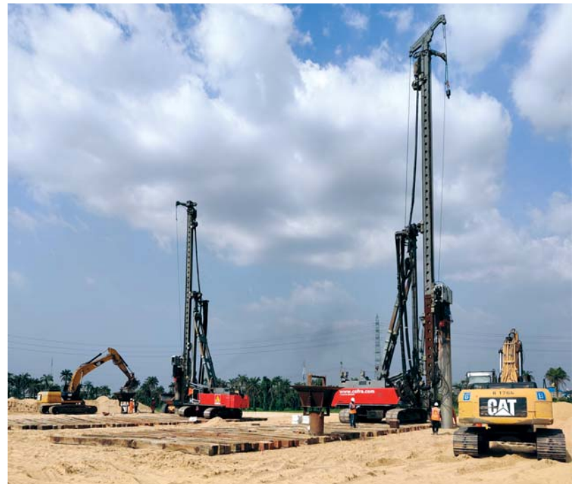
Figure 4 – Installation of Prefabricated Vertical Drains (PVD) to accelerate consolidation of the soft layers and limit residual settlements.
