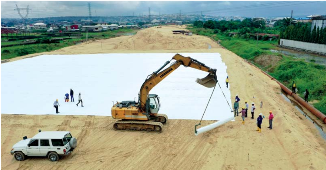
Figure 2 – Installation of high strength basal reinforcement.
