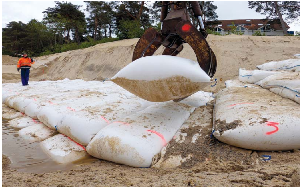
Figure 4 – Exact and stable positioning of the Geotextile Sand Containers of approximately 1.4 ton/element using crane clamping.
