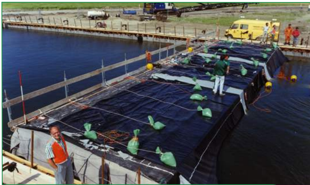
Figure 4 - Special pontoon for storage and launching the geomembrane to the water level
