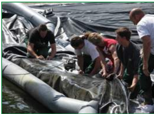
Figure 7 - Sealing of the major geomembrane with hot-wedge channel welding techniques on site before submerging
