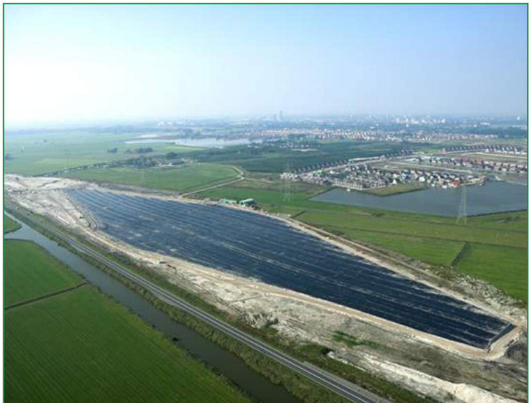
Figure 2 - Geomembrane in open excavation before submerging (Aqueduct RW31 Langdeel, 2008)
