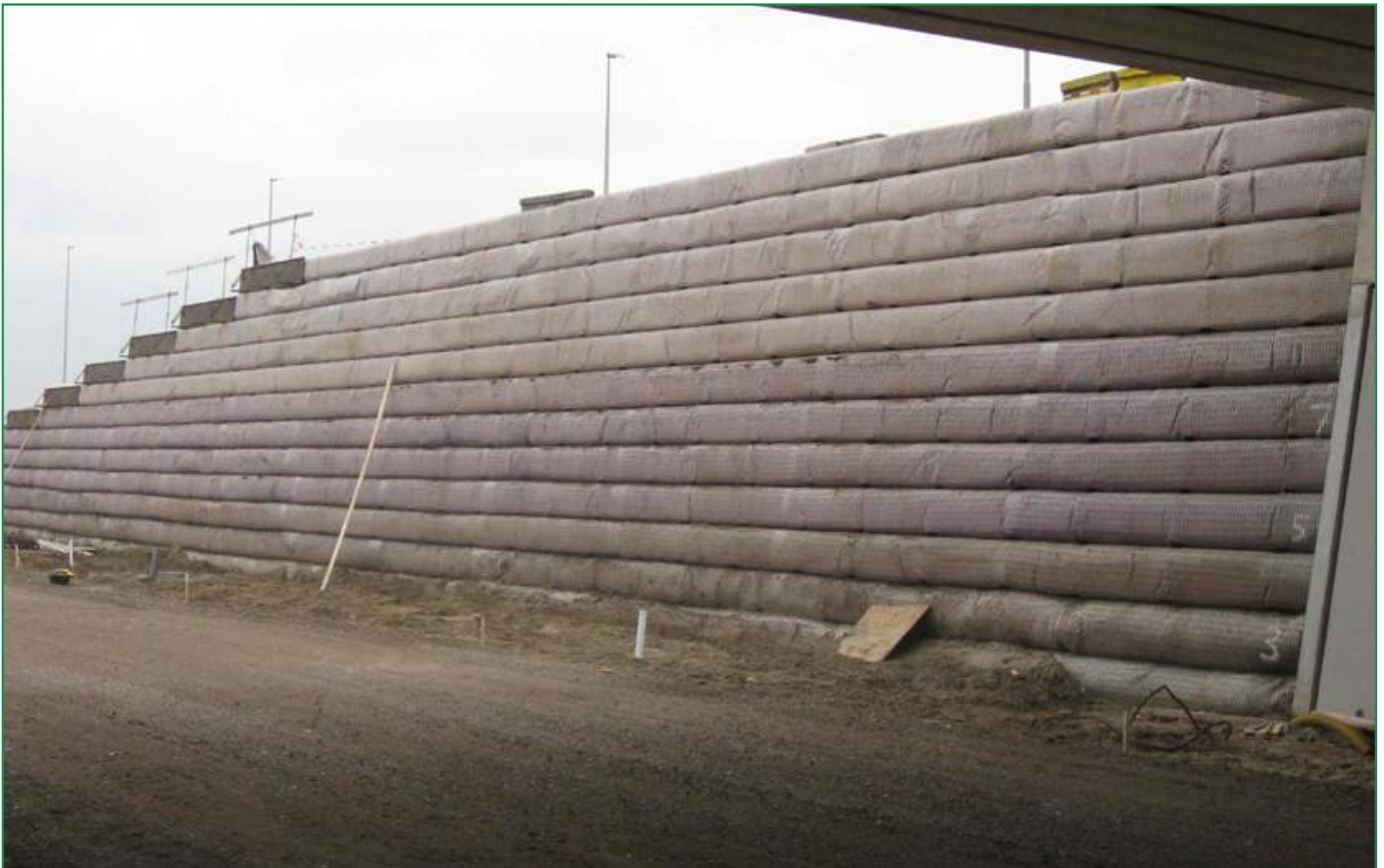
Figure 3 - Steep slope construction motorway A2, Utrecht 2011
