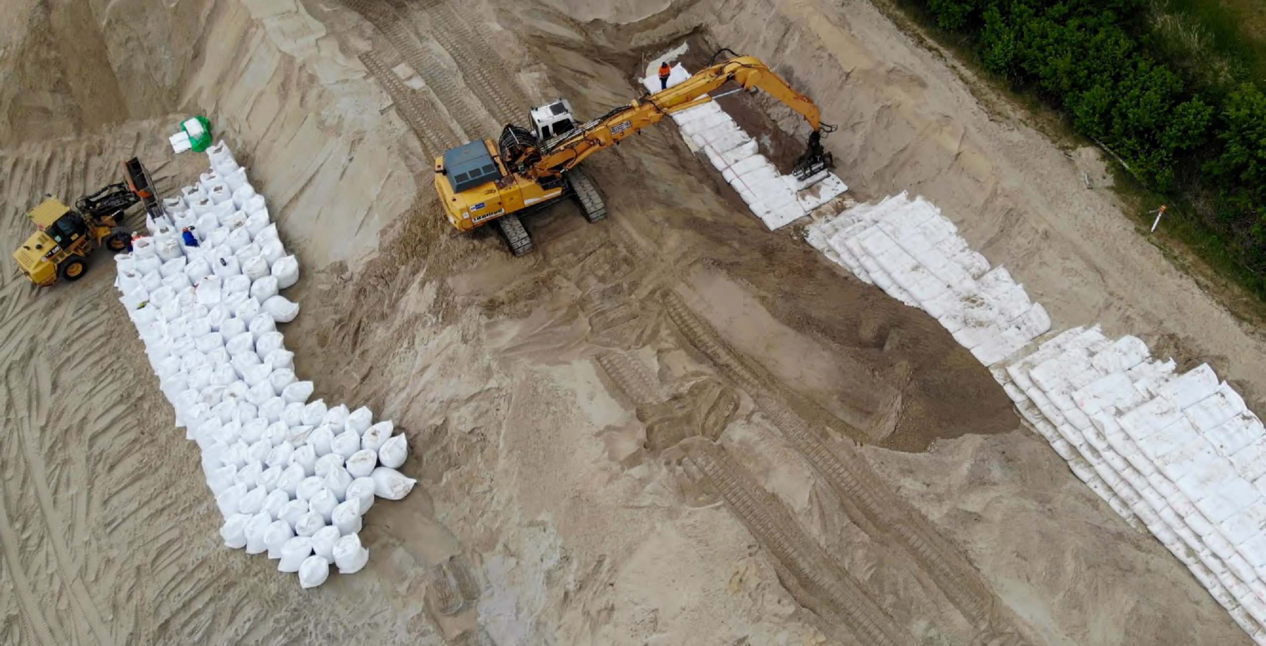
Coastal protection Ludmin, Mecklenburg-Vorpommern, Germany Solution with Secutex® Soft Rock - Geotextile Sand Container as beach wall protection structure
