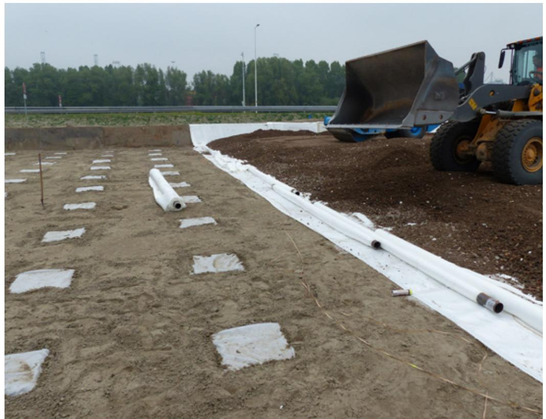
Figure 2 - Piled embankment for the A15 constructed with high strength woven geosynthetics.
