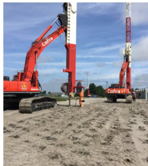
**Figure 1 -** Example of GPS based installation of PVD without the use of pre marking on the ground.
