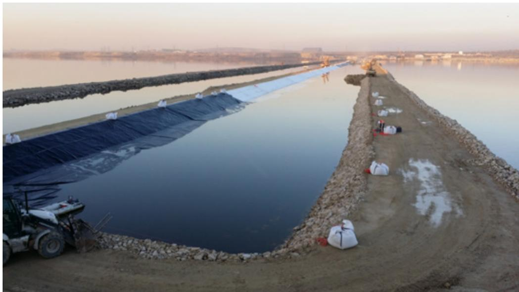
**Photo 1 - The installation of the geo-membrane at Lake Boyuk Shore**
