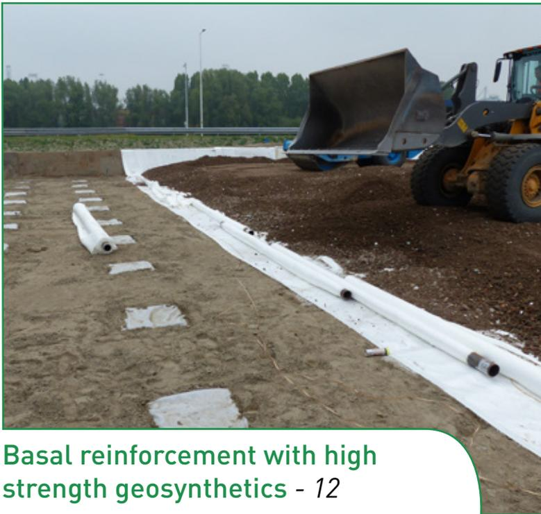
Basal reinforcement with high strength geosynthetics - 12
