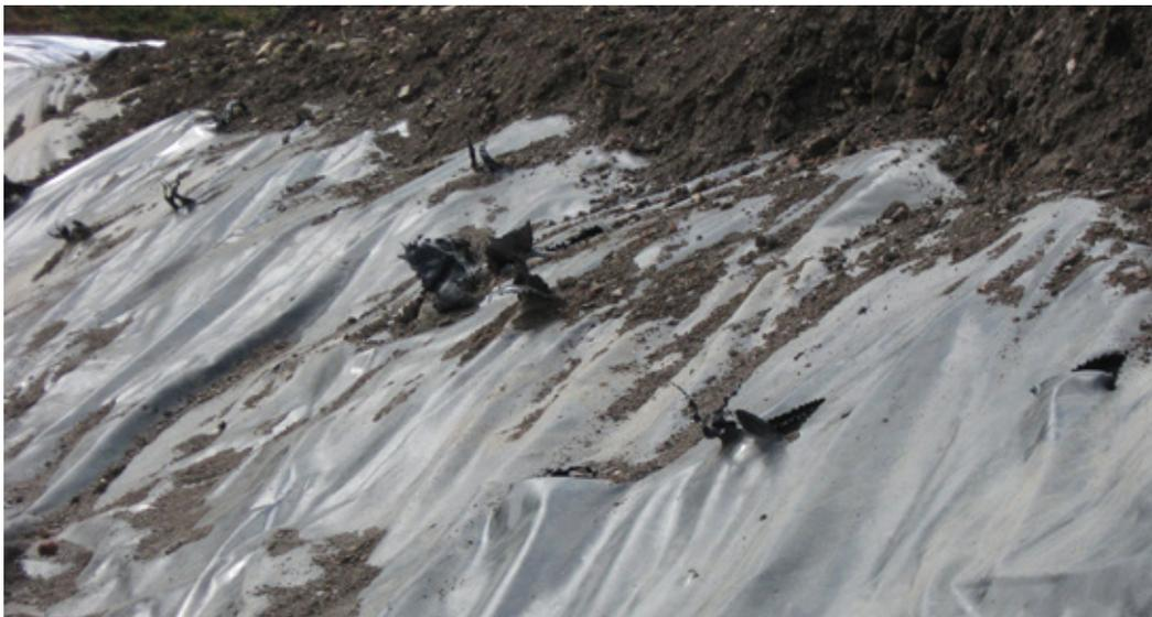
**Figure 7** - Mechanical damage to a geomembrane anchoring trench by using wrong backfilling equipment (crane) and less instructed personnel on site [Gerritsen]
