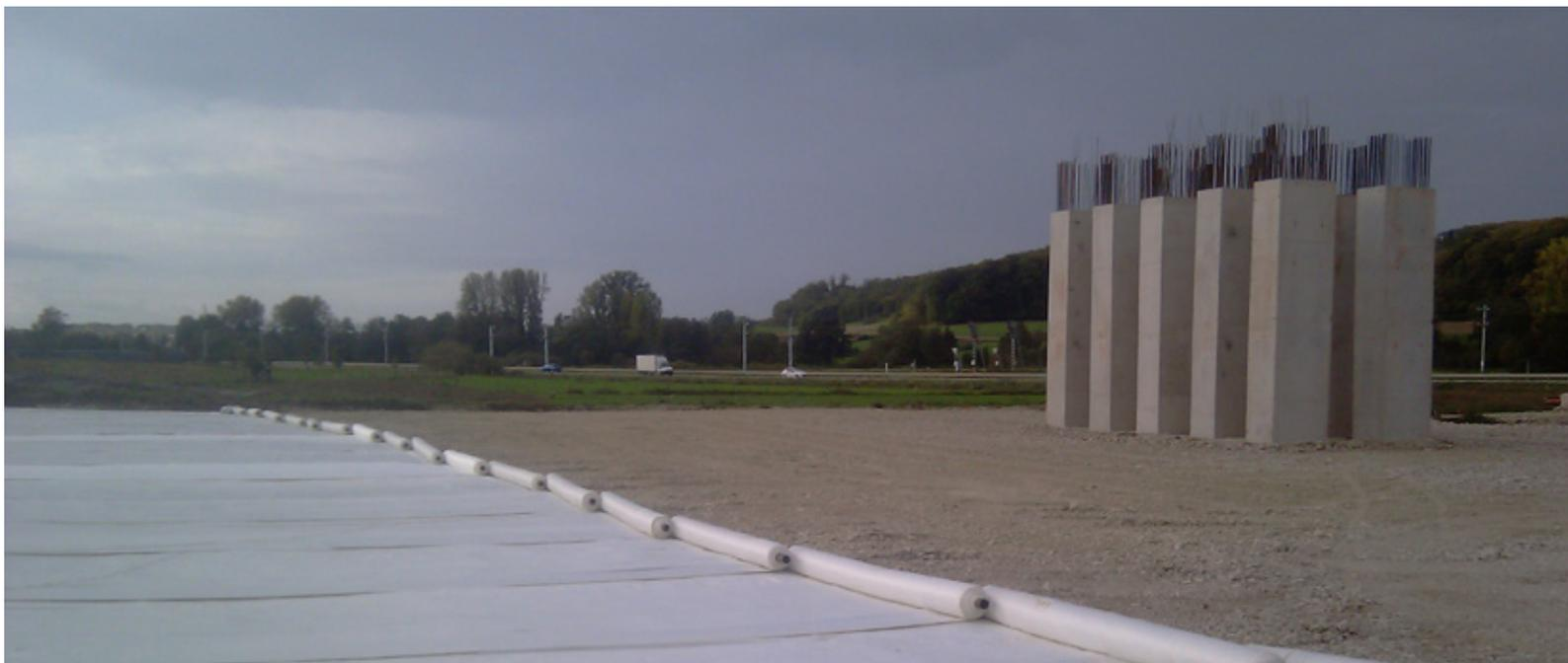
**Figure 3** - High strength woven geosynthetics preventing possible damages to a high speed train line in a French cavity-sensitive area.
