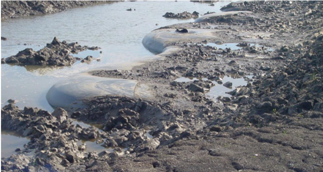
**Figure 6** - Geomembrane 'whales' due to uplifting water pressure below the geomembrane related to improper backfilling levels [Genap]
