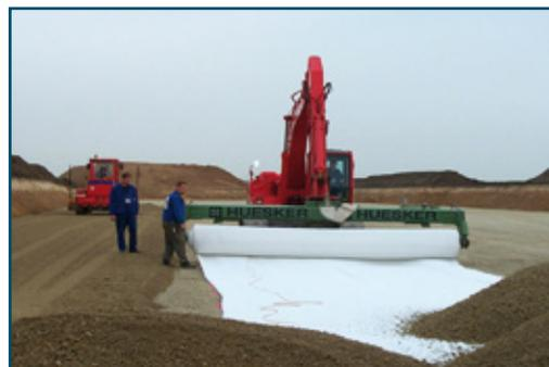
Base reinforcement: Stabilenka® geotextile
