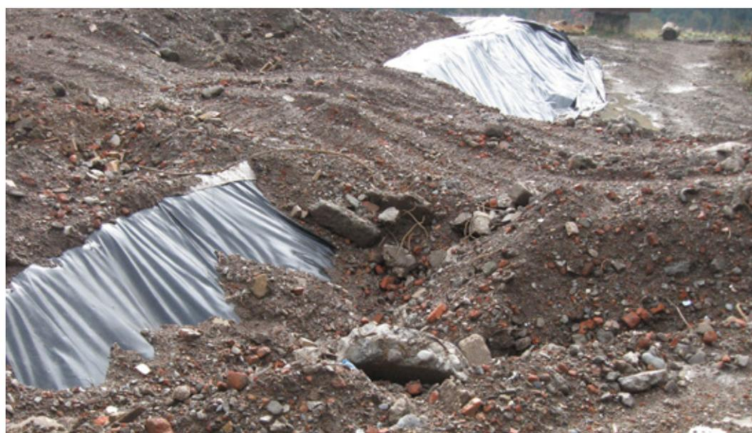
**Figure 4** - The presence of sharp/big stones without protective geotextiles will significantly increase the risk on damaging the geomembrane [Gerritsen]
