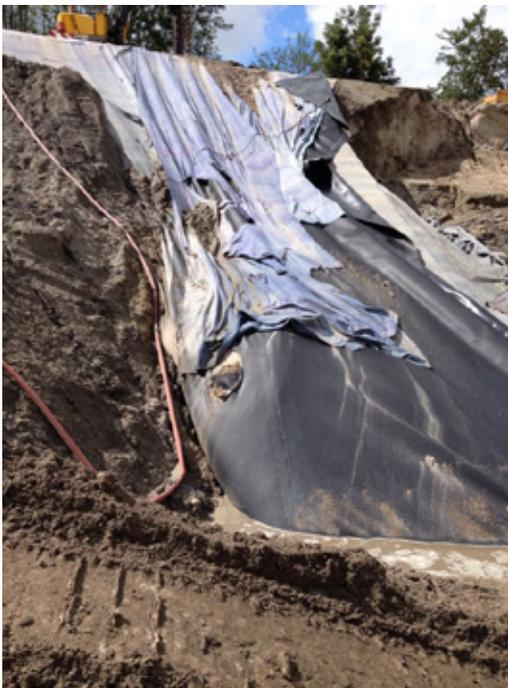
**Figure 1** - Slope failure by stability problems after finishing the geomembranes caused by external water pressures versus insufficient backfill levels [Genap]
