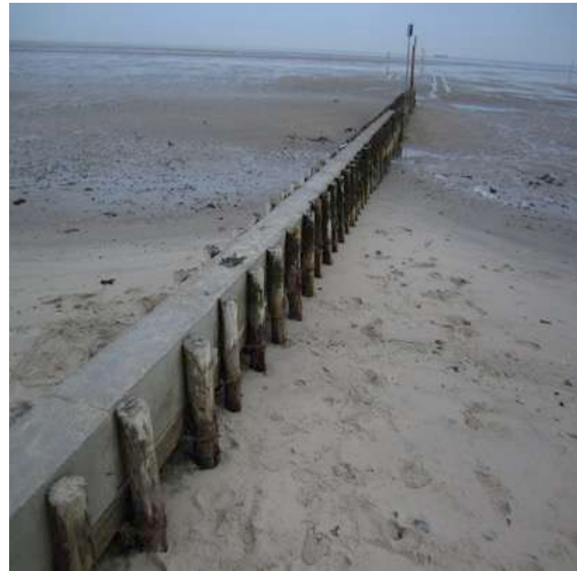
Groins as a combination out of wood and concrete
