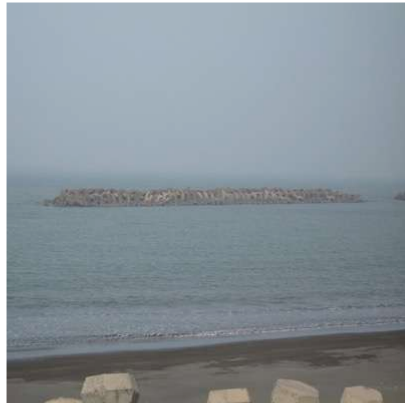
Breakwaters consisting of armor units
