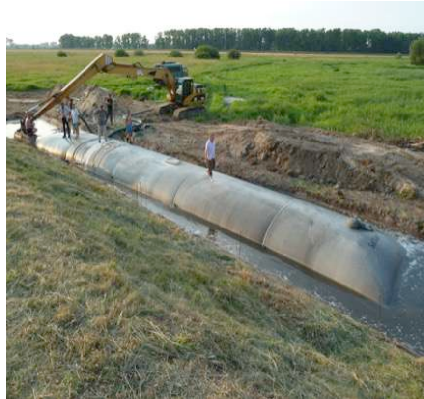
Installation in the dry
