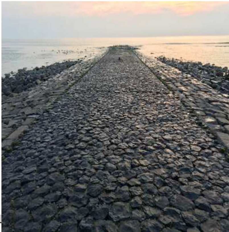
Groins made out of rock
