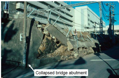
1995 Kobe Earthquake, Kobe line (railway)
