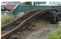
GRW with concrete facing and cement treated gravel directly behind the wall
