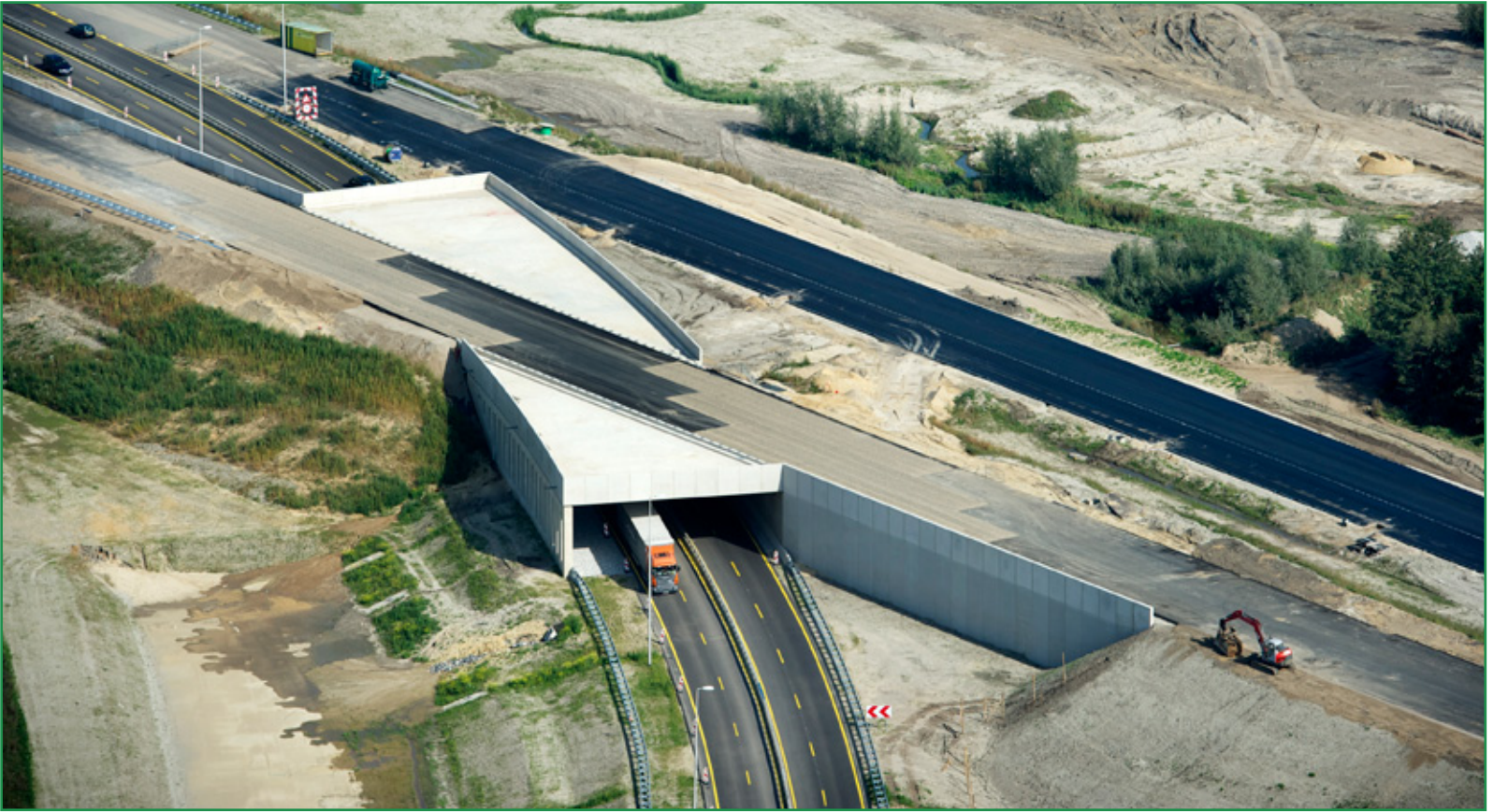
Figure 4 - Viaduct with "jointless" asphalt pavement construction. Venlo 2011
