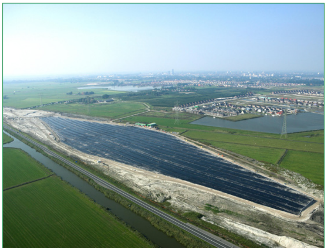
Figure 2 - Geomembrane in open excavation before submerging (Aqueduct RW31 Langdeel, 2008)
