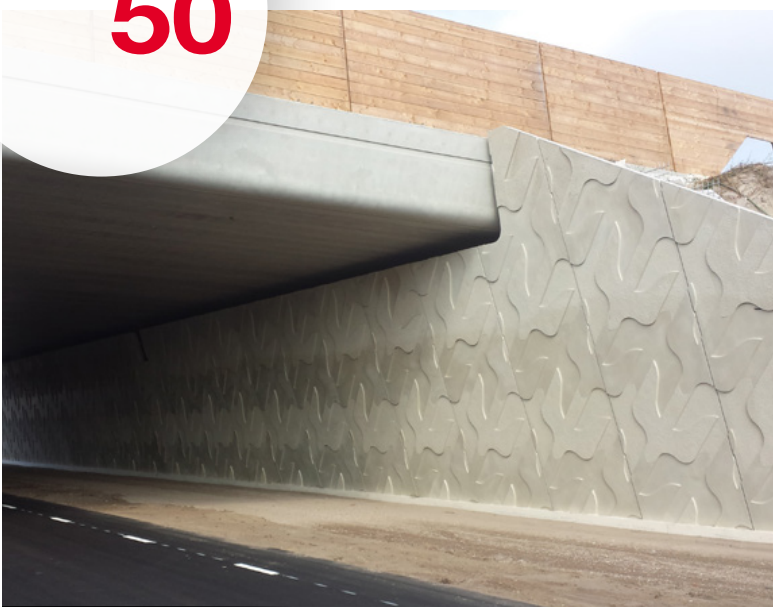
Weert Ecoduct - The Netherlands
