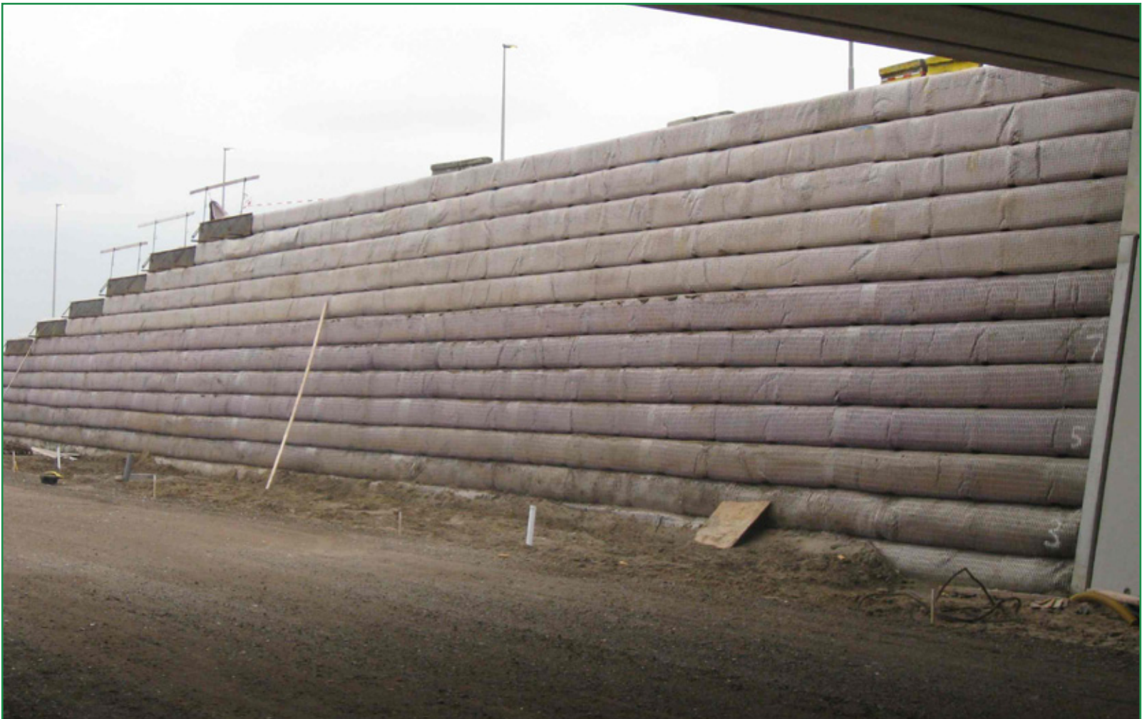
Figure 3 - Steep slope construction motorway A2, Utrecht 2011
