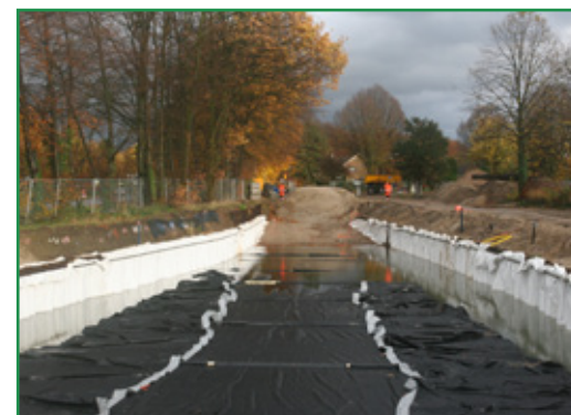
Figure 10 - Geomembrane U-polder in full construction before submerging (Deventer 2009).
