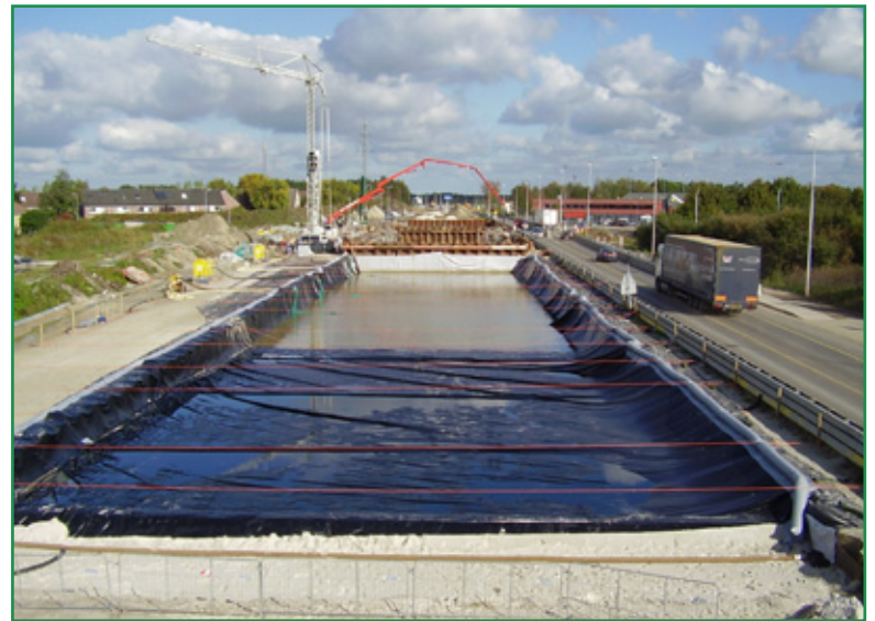
Figure 5 -Sheet pile polder, Assen 2008
