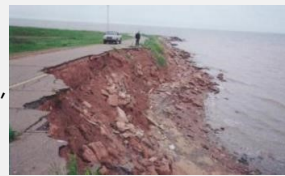
Severe slope erosion
